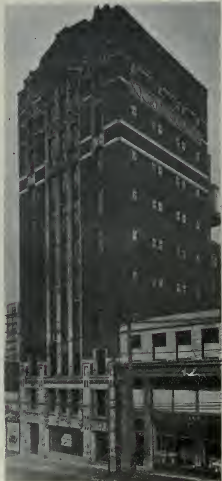
Fig. 3—The Southam Building, Bleury St.
